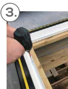
Secure the ring beam through the pre-drilled holes using the 70mm pan head screws supplied.
