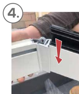
Position the Hip bar into the crown moulding and slide down to locate.
