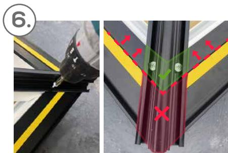
Place the frame (spider) into the ring beam, position and fix with 13mm pan head screws - AS SHOWN
