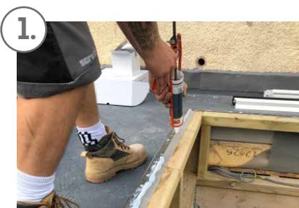
Apply suitable sealant to the perimeter of the kerb upstand.
