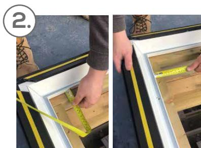
Place the ring beam on the kerb. Ensure it is square and centralise.
