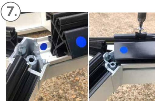
Position the ridge body with location dots at the same end. Attach with 80mm self drilling pan head screws.
