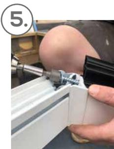
Secure the Hip to the moulding using 13mm Hex bolt and washer. Repeat for all hips.
